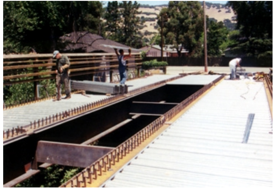
Once sections are installed, deck pan is added between the sections
