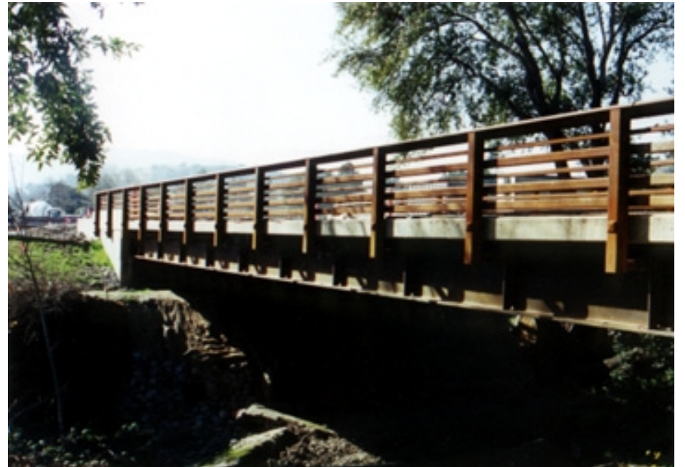
Finished Newspan® bridge built of A588 steel will weather to a deep patina over time
