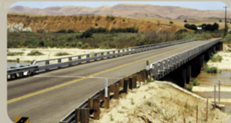
OUR LARGEST BRIDGE, 15 MATCHING RAILSPAN® MODULES WITH RAILING, 400' X 25'.
